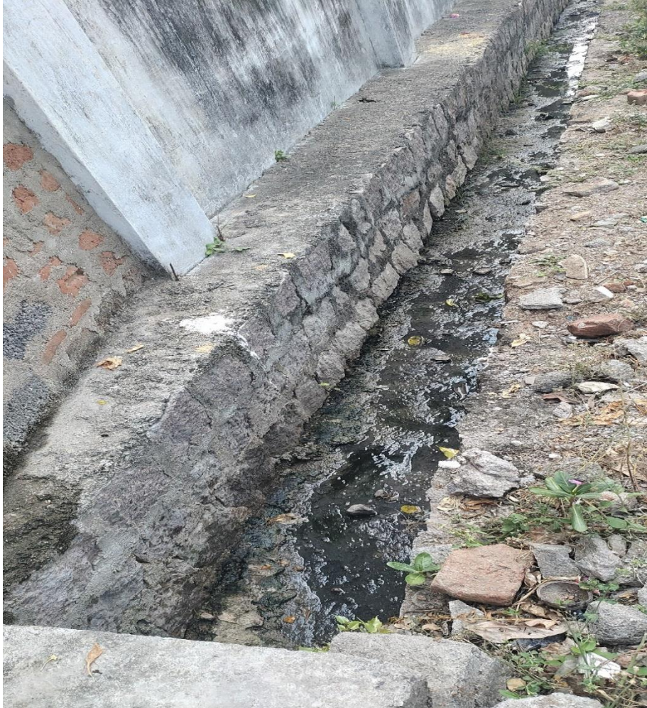
Picture 2: Stagnation due to rough bottom surface
